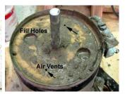
Remove the cylinder when you are comfortable that the concrete has cured sufficiently to be able to wire brush the teeth to expose the aggregate. Do not wire brush the V section of the teeth. Again, keep the end caps in place for about 24 hours until the concrete has cured enough to safely remove them without damaging the edges. Again, cover with a wet cloth and plastic and keep wet for curing.
