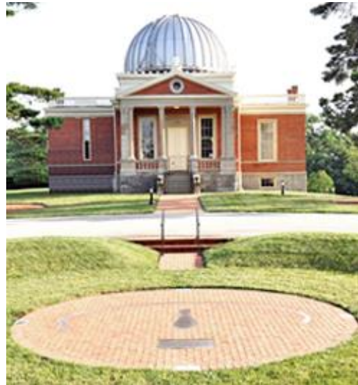
Precisely positioned brick, stone, and bronze make this Planispheric Analemma Sundial accurate to within 20 seconds and visible to all that visit the observatory. Image by L. Hite
